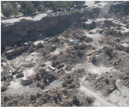
Figure 27. Collapse situation in Arg-e Bam collapse
