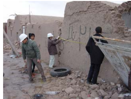
Figure 21. Survey of adobe masonry structure
